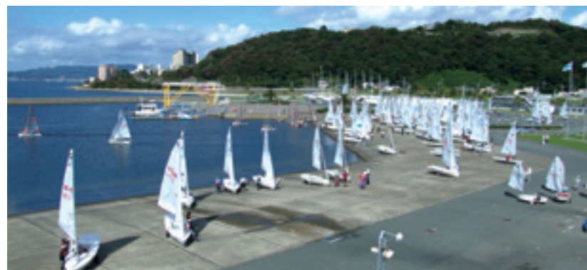
Slopes (2 slopes, total length 225.6 meters)
